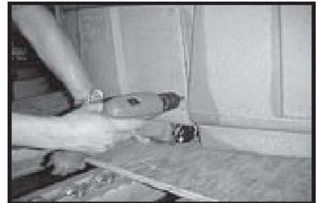
Remove & save access panel screws. Use caution when reinstalling the screws. Do not overtighten.
